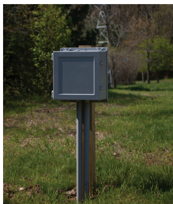
Pole mounted fiberglass enclosure for typical SSD
