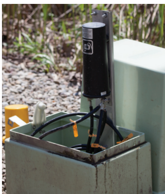
A typical SSD in a fiberglass ground enclosure
